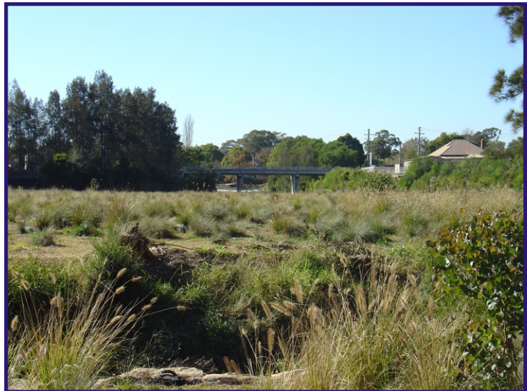
After - the floodway is constructed
