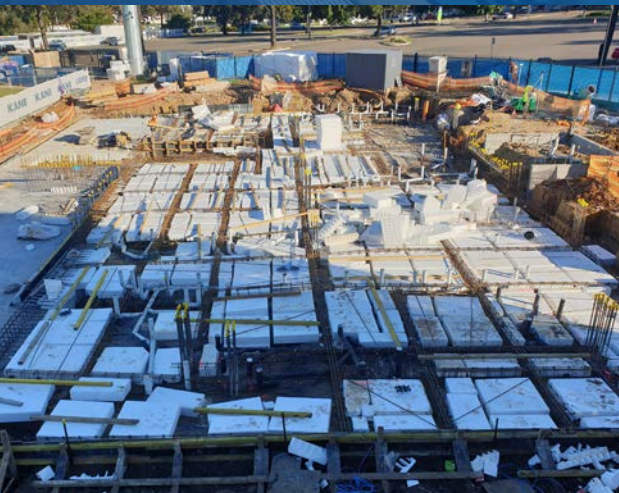
Work continues on the Fairfield Showground Pavilion
