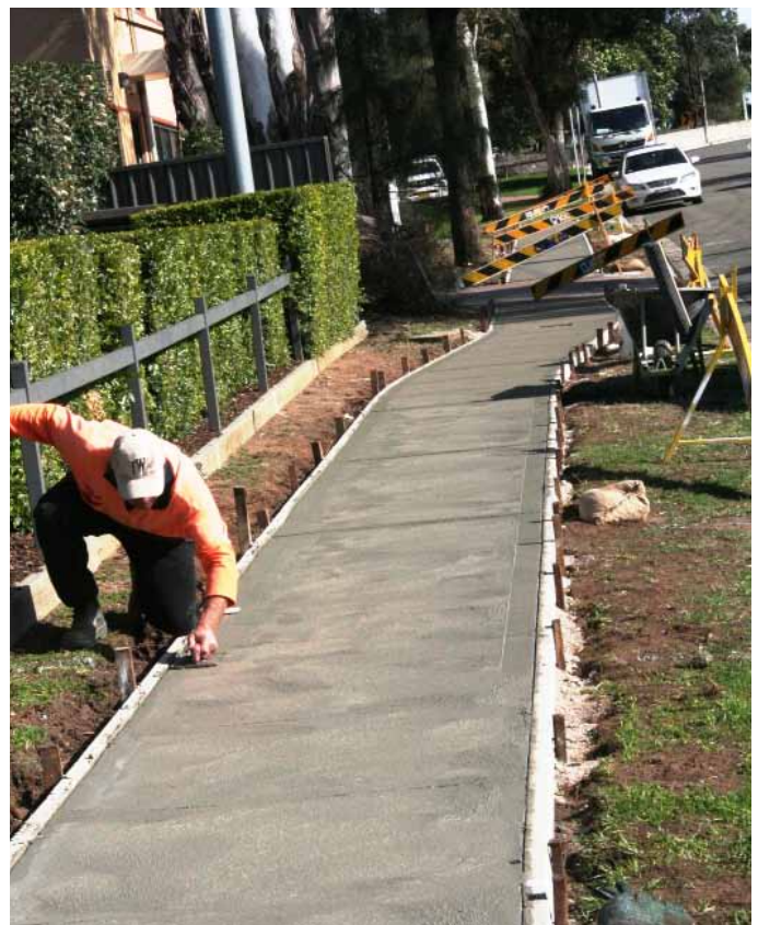
Construction of path paving at Daniel Street, Wetherill Park
