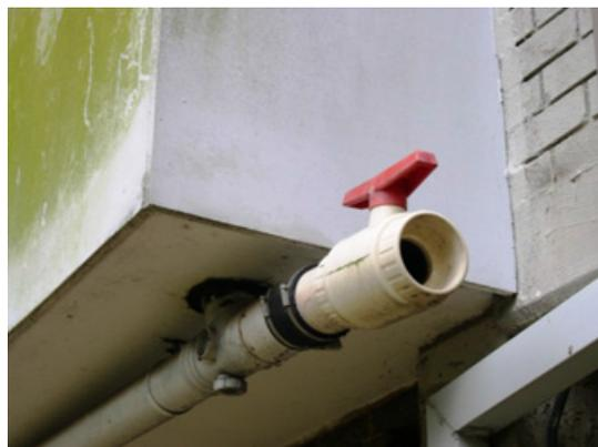
*Examples of floodproofing measures undertaken in Sandal Crescent include flood gates and enclosed balconies with stop-valves on drains to prevent intrusion of floodwater. Experience has highlighted issues related to maintenance of these facilities and maintaining the awareness of the occupants of the building of what needs to be done should a flood occur.*
