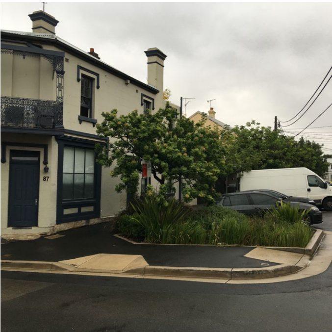
Water sensitive urban design basin integrated into street parking and footpath
