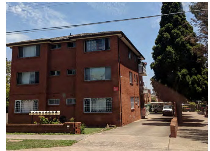
Figure 14 - Example of a 1960's walk up development in Cabramatta Place
